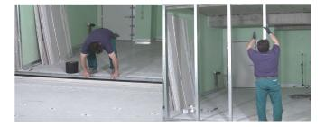
Cover the insulation layer by screwing the second gypsum boards on the metal studs
