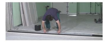
Fix the gypsum boards on one side. Insert the Fybro panel
