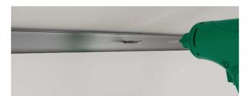
Fix the metal stud to the acoustic bracket
