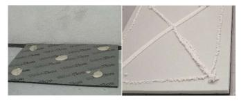
Fix the gypsum board with the glue and/or appropriate screws
