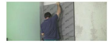
Apply the plastic mesh tape in the gypsum boards jointing lines. Grouting
