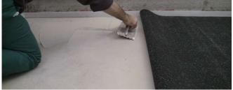
Spread the bi-component concrete glue, layer the ceramic tiles over the adhesive glue
